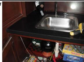
7. Faucets/Traps: Delta fixtures with a metal trap - At the kitchen sink the hot and cold operation is reversed.
