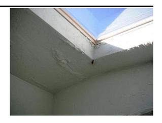
20. Walls: Paint and tile - Some minor wall damage noted from moisture intrusion near the bay window in the dining room.
