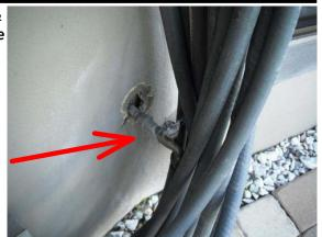
10. Lawn Sprinklers: Front and back yard - The lawn sprinkler system has broken heads throughout and there appears to be a broken line on the east side of the home, once the system is fully repaired it will need to be tested and adjusted so that no water is spraying onto the home.
